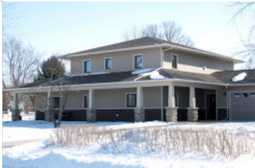
The Stanton House in Urbana, Illinois, built in 2008, has 2,200 ft 2 of floor space (as calculated in PHPP), R-64 walls, R-87 roof, R-51 sub-slab insulation, and triple-glazed windows rated at U-0.17 (0.96 W/m 2 K).
